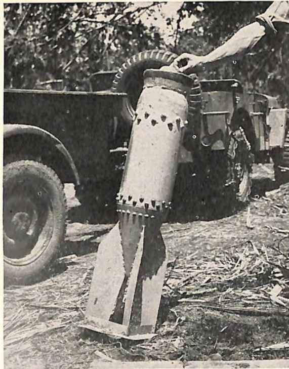
Figure 69. Model 99 (1939) 63 Kilogram General Purpose H. E. Bomb.
